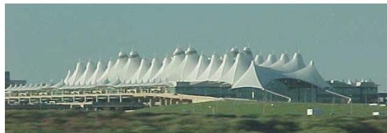
Denver International Airport
