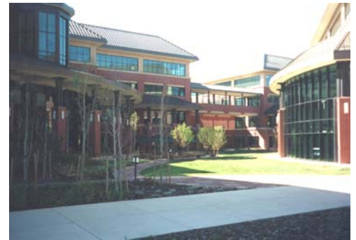
Level III Communications Complex
